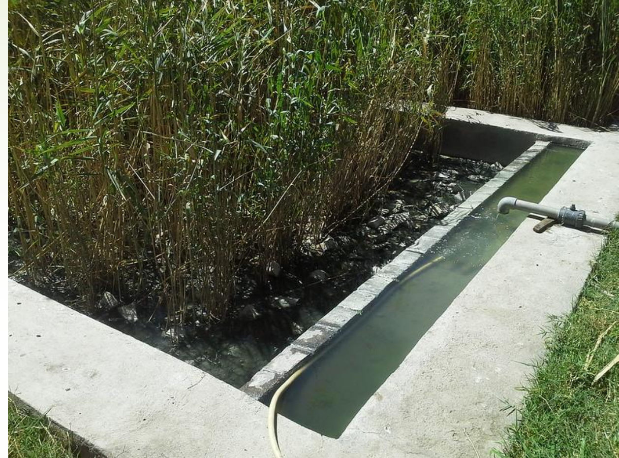
© Constructed wetland at the Modjo Tannery at Modjo" Bio-Innovate-ILRI/Albert Mwangi https://creativecommons.org/licenses/by-nc-nd/2.0/deed.en
