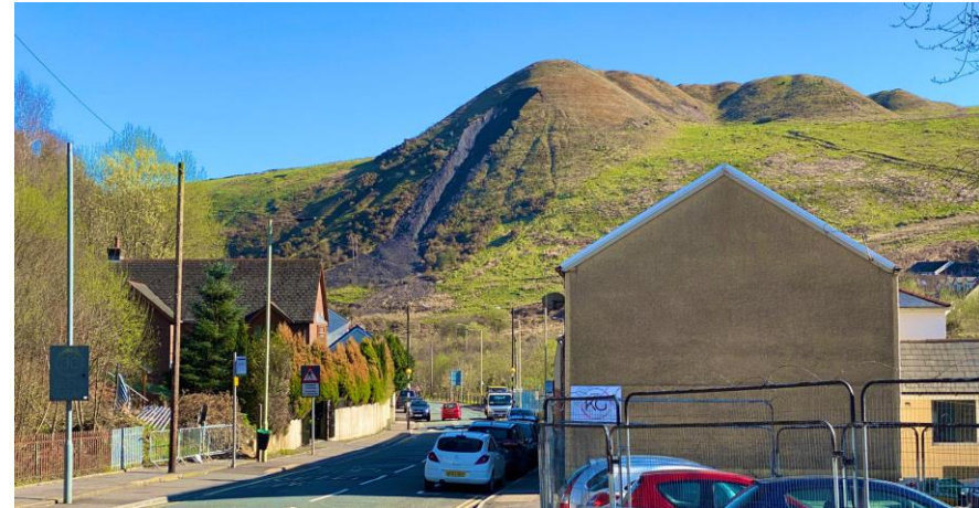
A small failure in a coal waste tip in South Wales. (Clear South Wales's Coal Tips).
